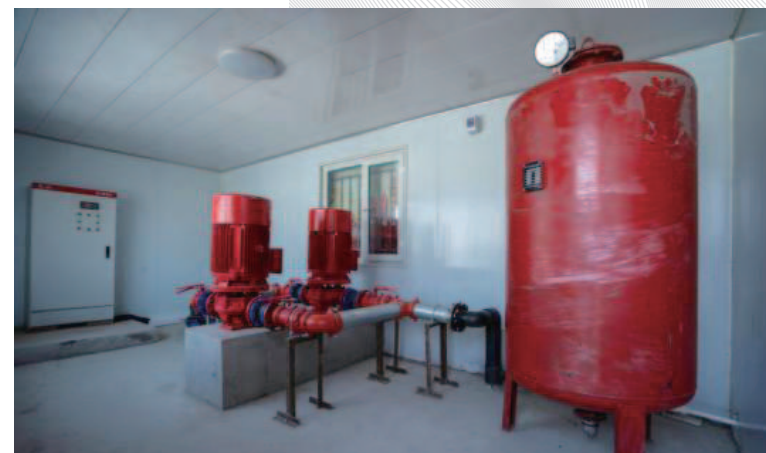
Rainwater collection system
