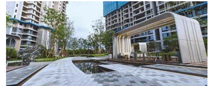
Exterior workshop — façade and landscape construction
